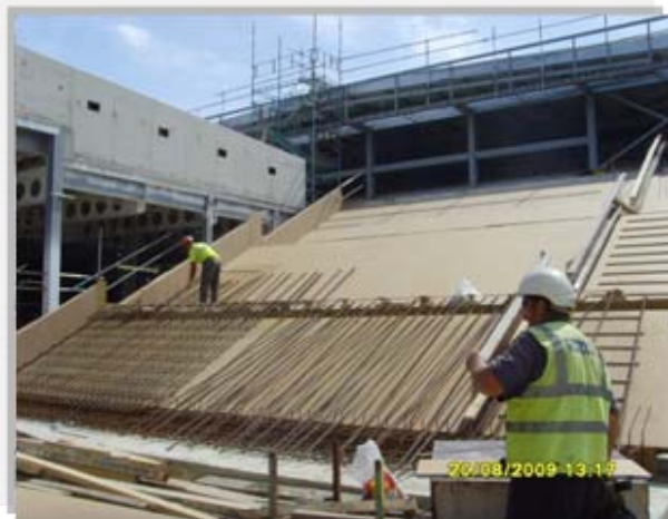
Amphitheatre under construction
